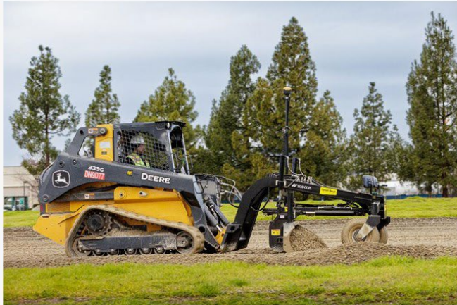
Addition of two systems using GNSS and surveying instruments
