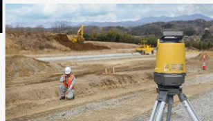
Layout Navigator LN-100 at Construction site
