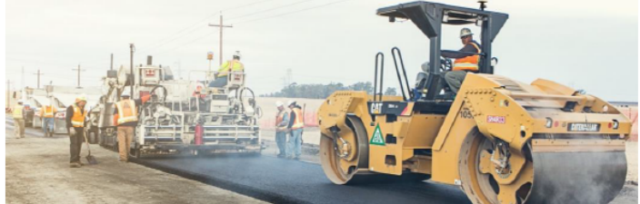
Photos of IT construction at road construction sites
