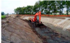
Emergency measures such as building levee, excavating river channel
