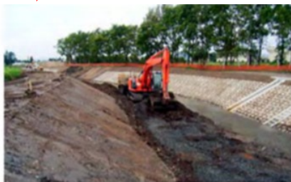
Emergency measures such as building levee, excavating river channel
