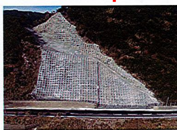
Emergency measures such as reinforcement of road slope protection
